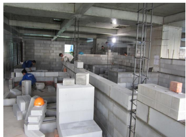
Placement of bricks (AAC)
